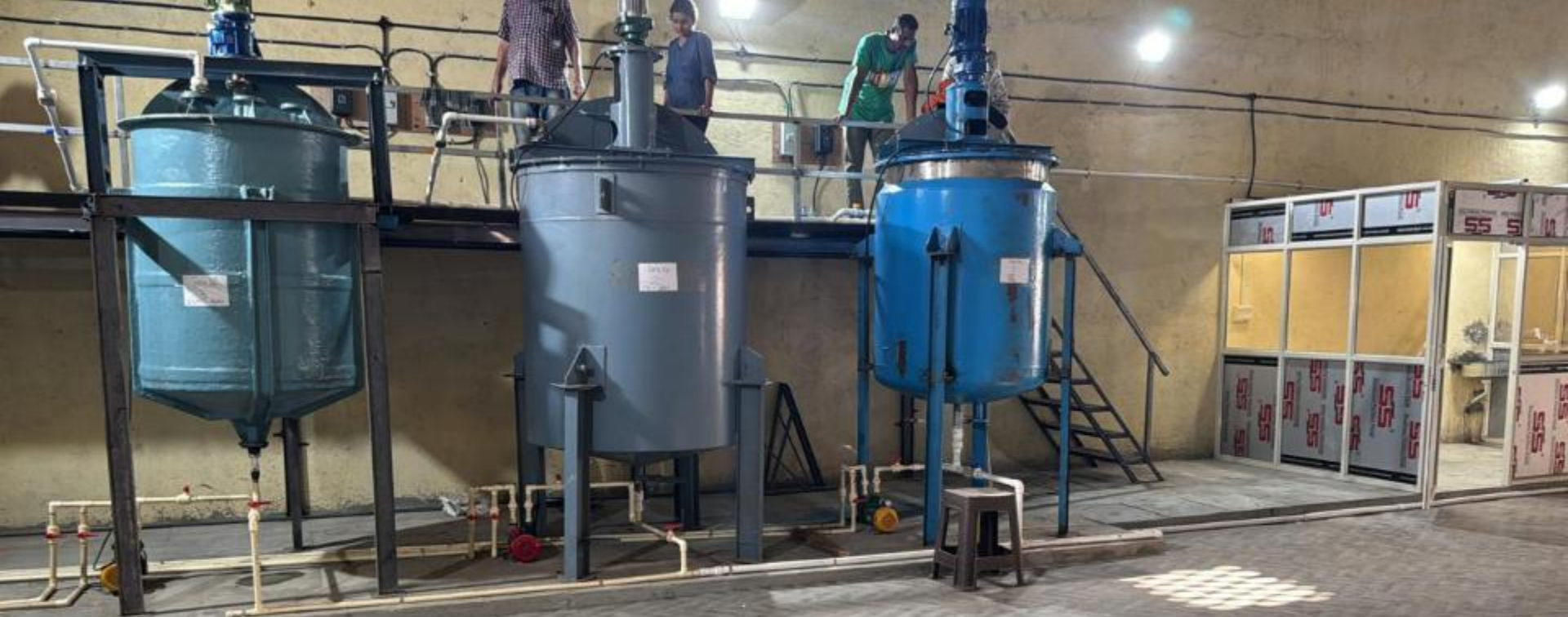
Panoramic view of the local production plant facility in the Maharashtra region of India
